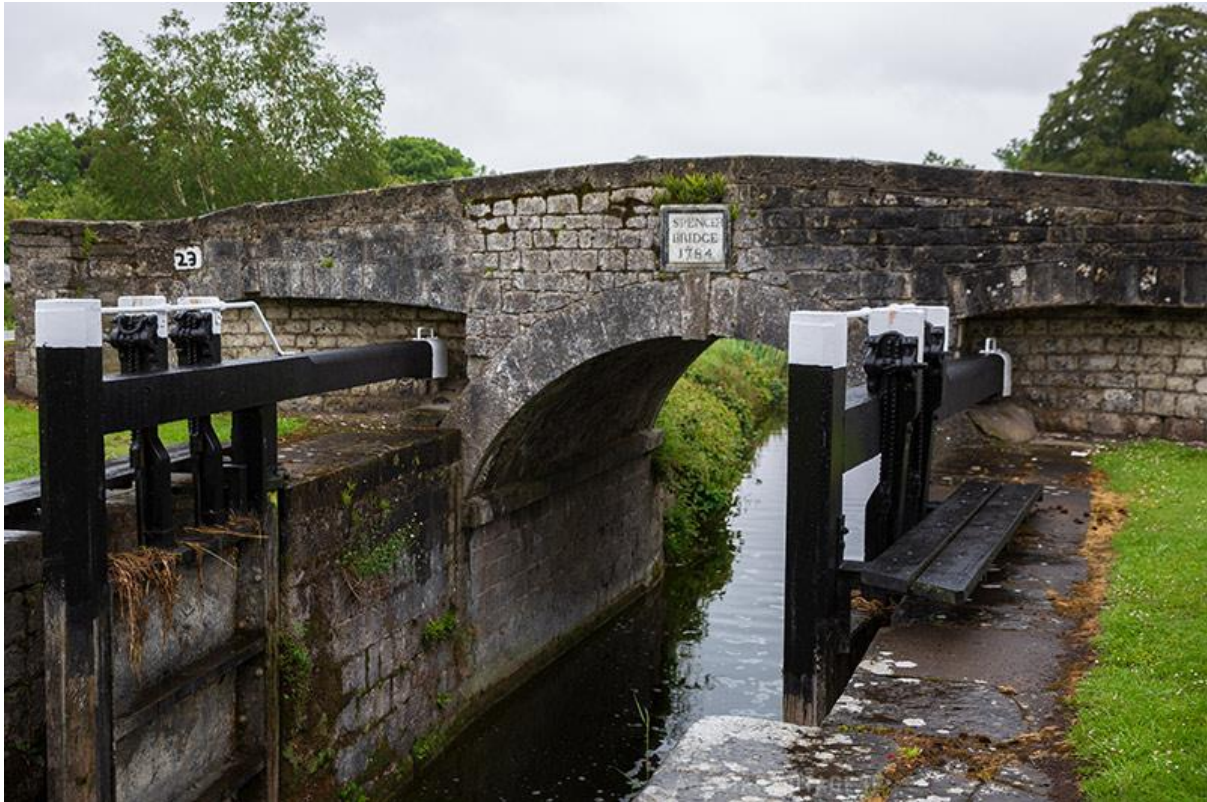
Figure 17: View of Spencer Bridge, Rathangan
